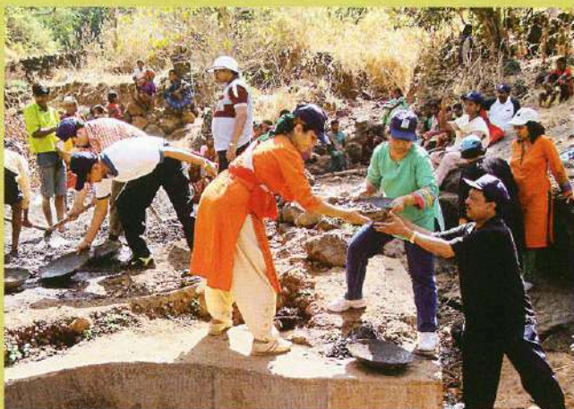
Villagers and BPCL employee volunteers working together on bund construction
