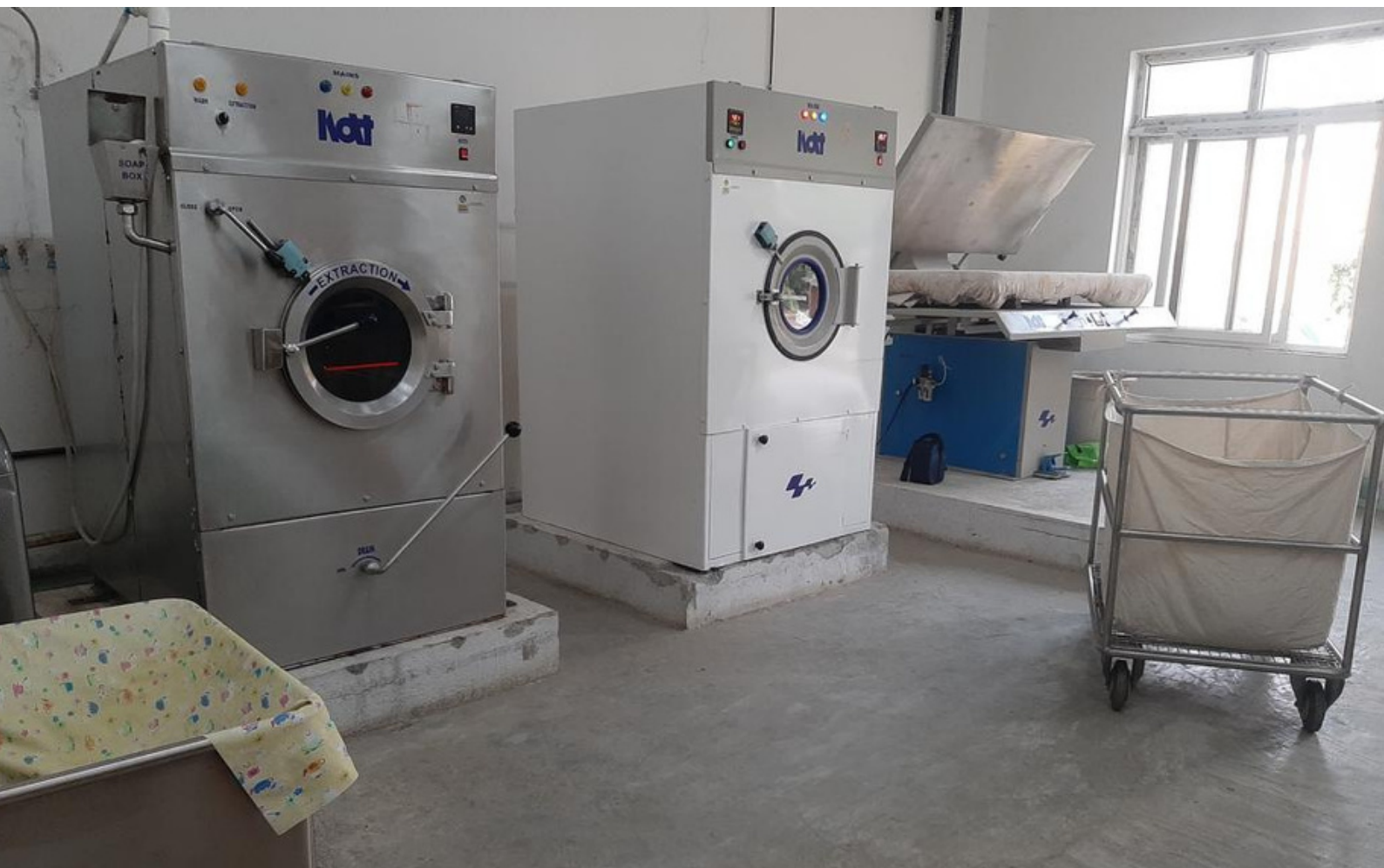
Machines in Laundry Department to Sterilization of Linen and clothes of staff and patient
